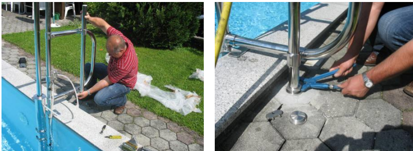
Fig. 3.8 - Insert the additional support and screw it to the console using the cap nut.
