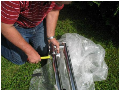
Fig. 3.3 - Adjusting the protrusion of the pool edge at the spacer
