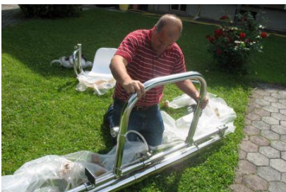
Fig. 3.5 - Attaching and screwing the C-tube
