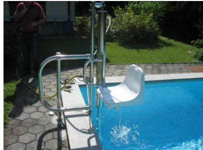
Fig. 3.13 - Checking the immersion depth and entry height
