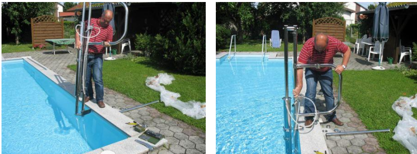
Fig. 3.7 - Placing the pool lift at the edge of the pool
