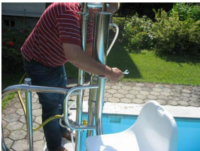
Fig. 3.12 - Tightening the seat bracket
