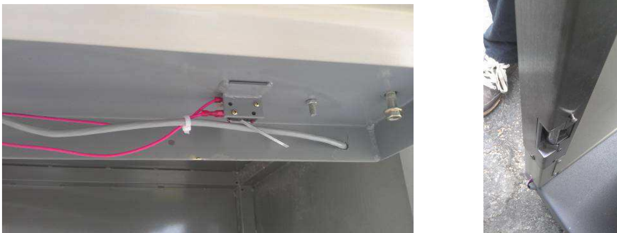
Fig. 3.21 - Pull in the connection cable
