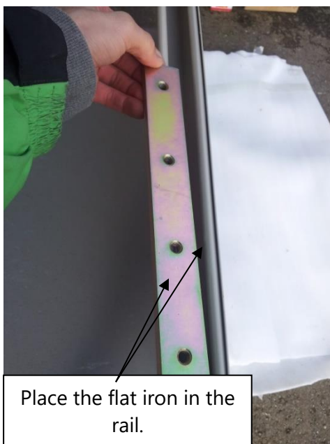
Fig. 3.11 - Place the flat iron in the rail.
