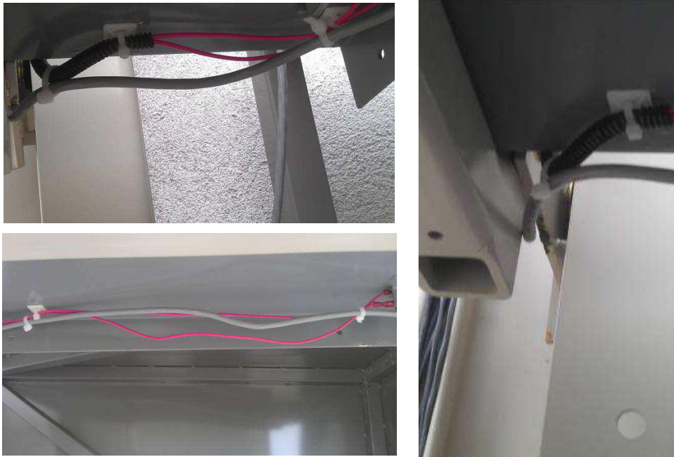
Fig. 3.20 - Laying connection cables
